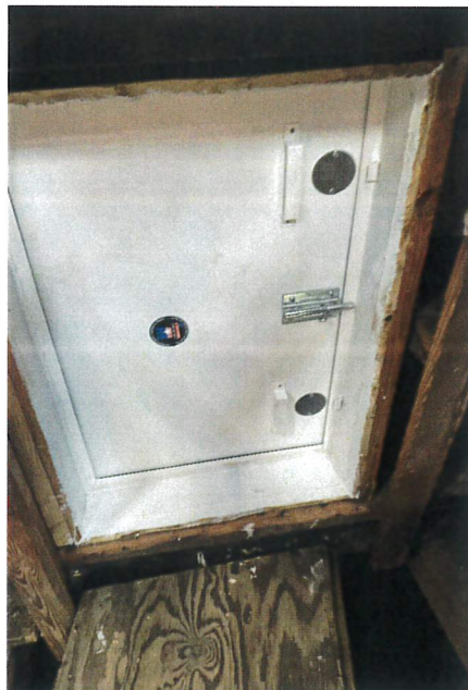
5 Completed roof door.
