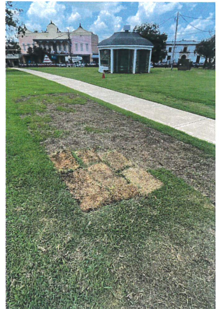
3 Sod to be replaced.
